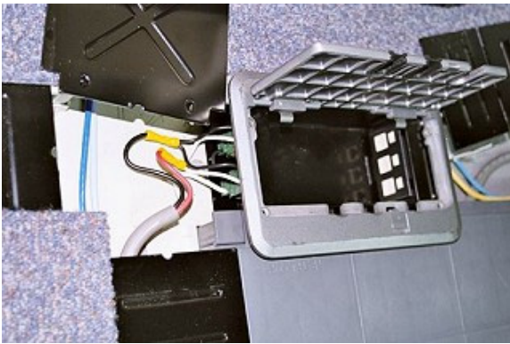
SB603 accommodates 2 X 110 volts power sockets and 3 X Cat. 5 or Cat. 6 data jacks. SB403 accommodates 2 X 110 volts power sockets and 2 X Cat. 5 or Cat. 6 data jacks.
