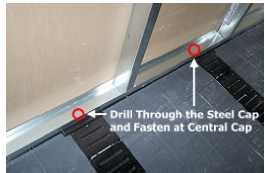
In case the partition lays on Cable Trench, drill at floor track and steel trench cap, fasten by < 15 mm length self drilling screw.
