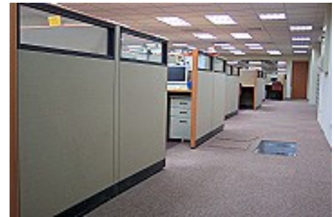
Half-height partition on ECO series power, data, voice cables distributing under the floor, neat and no limitation.
