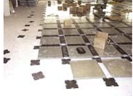
Installation of 40 mm and 50 mm height for office or school, renovation or new, where ceiling height is limited, and still provide large capacity for cable routing
