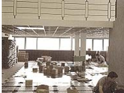
Installation of 40 mm and 50 mm height for office or school, renovation or new, where ceiling height is limited, and still provide large capacity for cable routing
