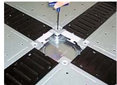
4 mm hex-key wrench to adjust height
